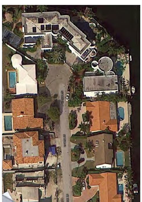
HOUSE 4 (Roof top Terrace)
